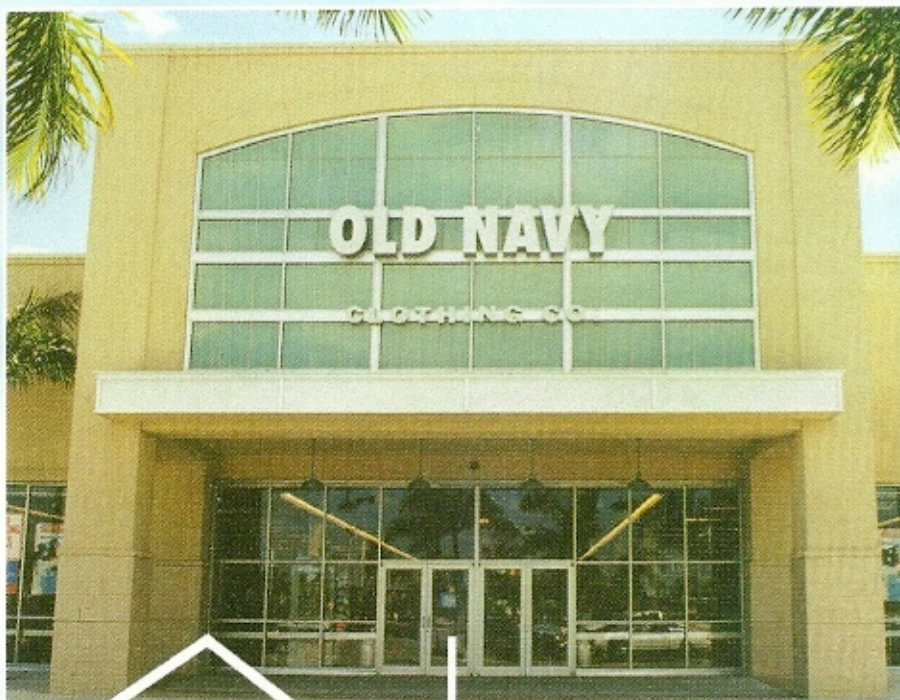
OLD NAVY STOREFRONT, PEMBROKE PINES, FL USA
